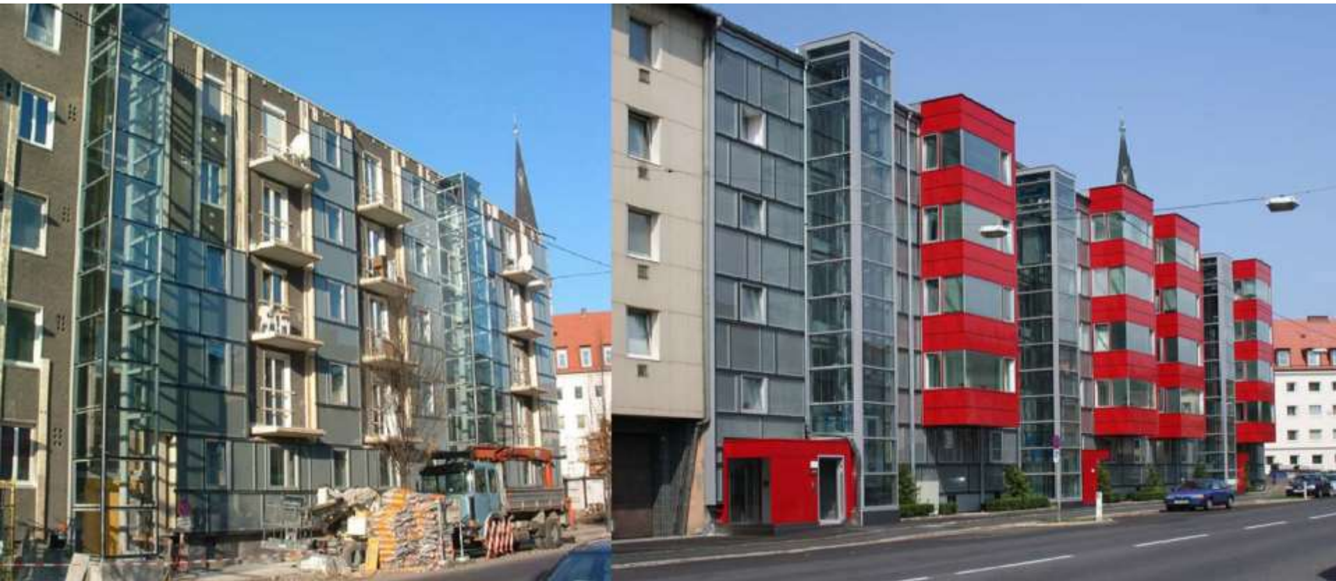
Austria- Linz, dwelling renewed to reach passive house criteria (Arch+more)
